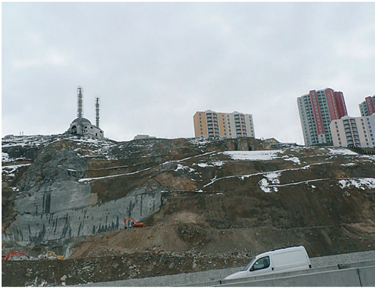
Figure 2: Tearing down the gecekondu for urban transformation Project (Source: Mendilcioğlu 2011).
