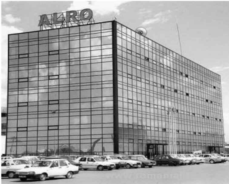
Figure 3. Registered office and corporate headquarters of the company ALRO S.A. Slatina.
