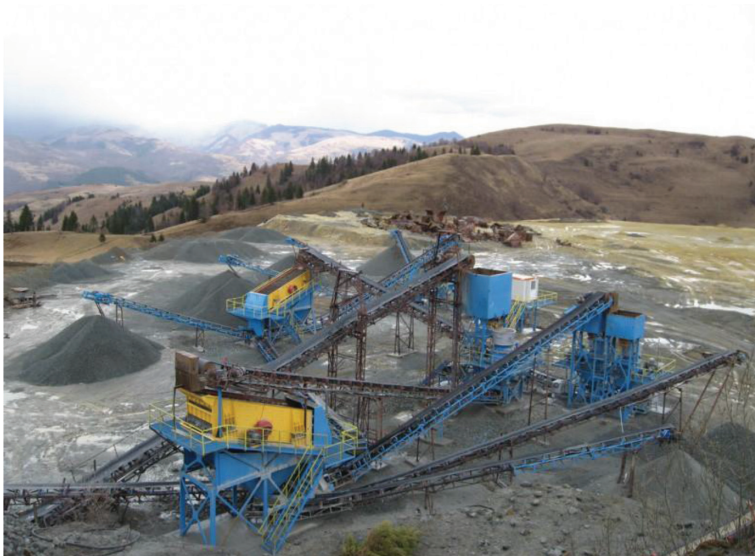
Figure 4. The processing plant of ores within CupruMin Abrud.
