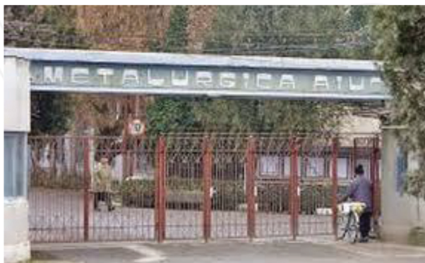
Figure 5. Access within the enterprise Metalurgica Aiud.
