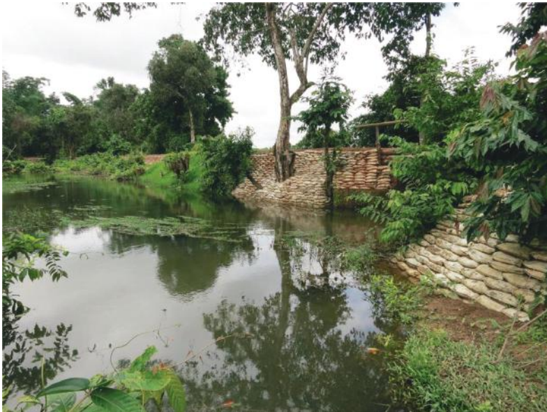
Figure 13. Road condition 1 year after the completion, during rainy season.
