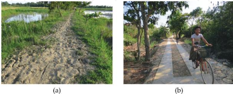
Figure 16. Road condition: (a) Before construction; (b) condition 1 year after the completion.
