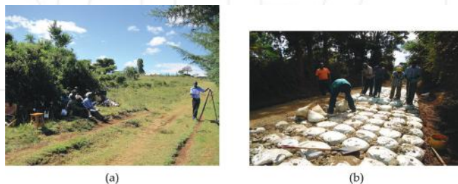
Figure 22. Training/demonstration of spot improvement using Do-nou technology: (a) Training at road side; (b) demonstration on Do-nou technology.
