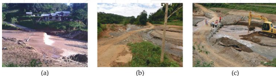
Figure 20. Vented ford affected by a typhoon and emergency work done by the provincial government: (a) Overflowing; (b) deposited sedimentation; (c) removing the sedimentation by the excavator of the provincial government for emergency.
