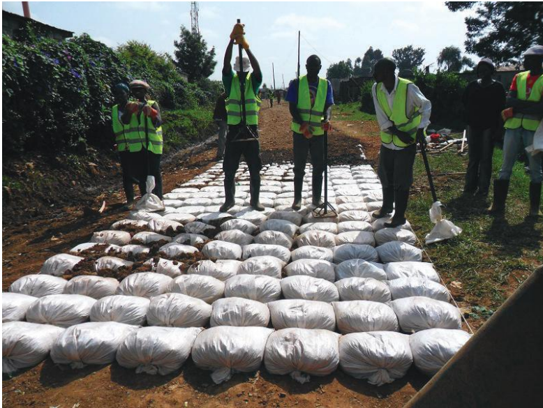
Figure 6. Practical manual compaction method for community work.
