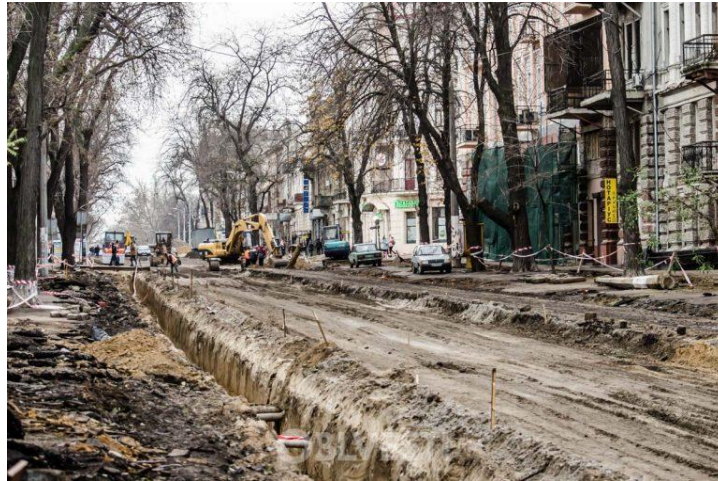
Pic. 8: Reconstruction of the Transfiguration Street in 2017
