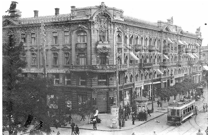
Pic. 3: Building "Passage" after the liquidation of the consequences of the fire
