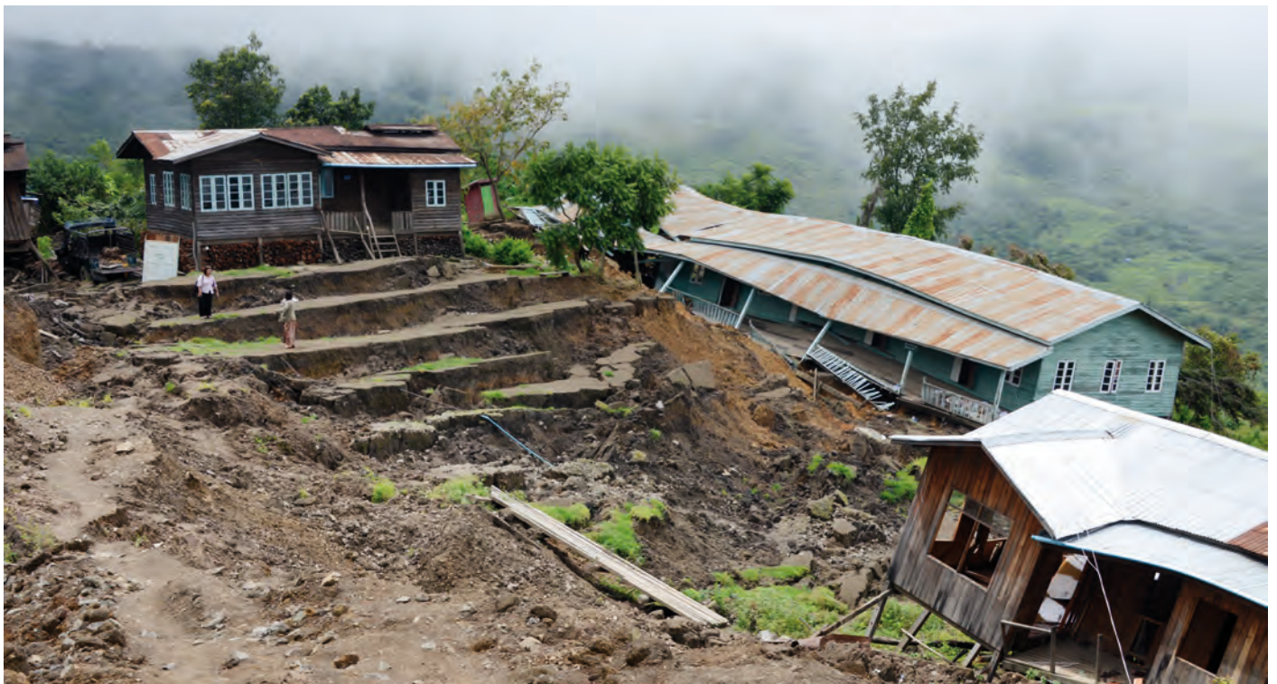
Step-like landslide in Hakha, Chin State in August 2015
