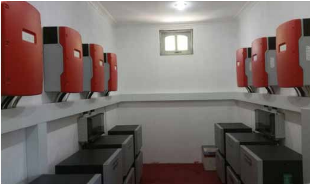
Solar photovoltaic array ( upper photo ), and battery bank and inverters ( lower photo ) in Dhihdhoo Island.
