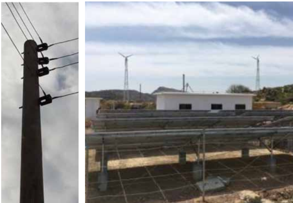
Concrete transmission pole at the Khushab site ( left ) and the solar PV–wind hybrid installation ( right ) at Khushab, Pakistan.
