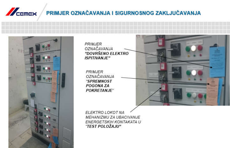
Figure 8 Example of marking and locking MCC drawer
