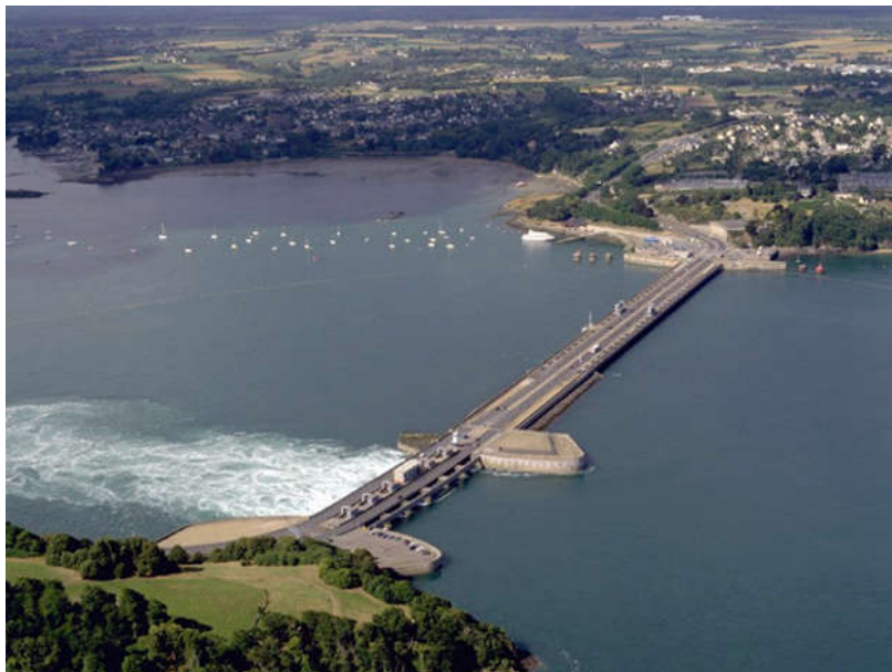
Figure 23 La Rance tidal barrage
