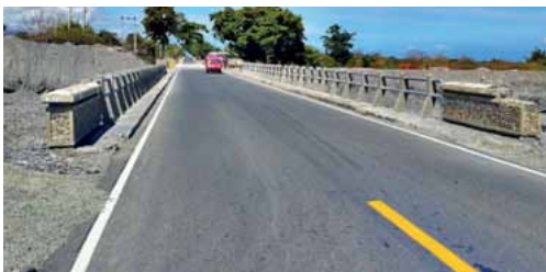
Top: Before construction, Liquica-Maubara road section; Bottom: Same road section after construction.
