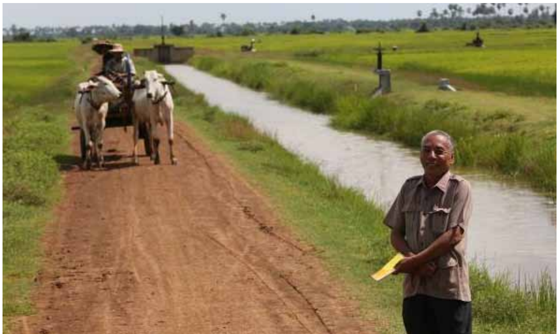
Reliable access to water. Su Ren, chief of Boeng Commune, stands proudly along the upgraded canal, which has boosted the livelihood and food security of farmers of the village.
