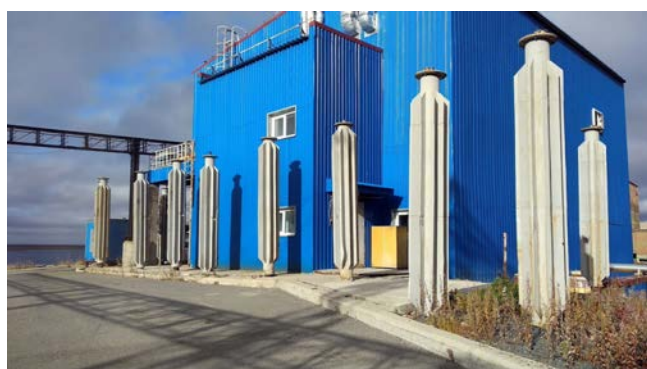
Figure 8.3. In Russia, thermosyphons are also often used to protect buildings, in combination with elevating structures on piles, such as with this building in the city of Dudinka (2018). Photo: Nadezhda Zamyatina
