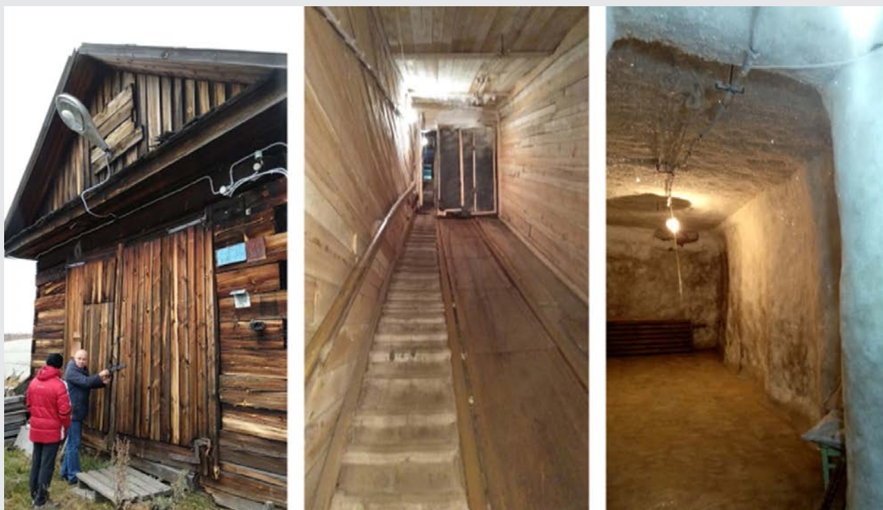
An entrepreneur in the city of Igarka (Krasnoyarsk Territory, Russia) demonstrates a natural refrigerator - a glacier (lednik), in which the permafrost cold was used to cool food. In the middle of the 20th century, in the chambers of this glacier, the annual supply of food for the city, imported during the summer navigation, was stored. However, in modern conditions, the glacier is not used, since the ability to maintain a constant temperature does not meet modern sanitary standards. Photo: Nadezhda Zamyatina
