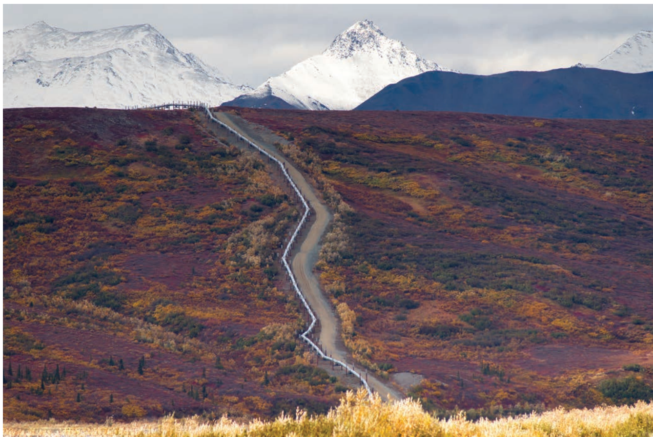
Trans-Alaska Pipeline. Photo: Colourbox
