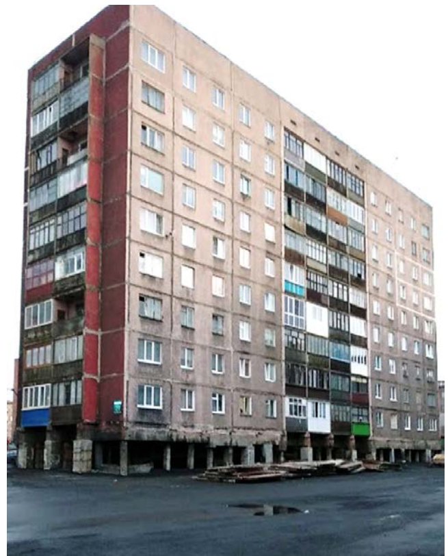
Figure 8.1b. The elevation of buildings (and other infrastructure) onto pillars allows for a ventilated layer between the structure and the ground, which helps protect against permafrost degradation: Norilsk, Russia. Photo: Nadezhda Zamyatina.
