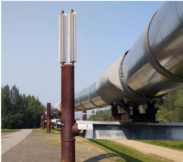
Figure 8.2. Thermosyphons alongside the Trans-Alaskan pipeline draw heat out of the ground and help keep permafrost temperatures low enough to support the above-ground structure. Alaska pipeline (2019). Photo: Nadezhda Zamyatina
