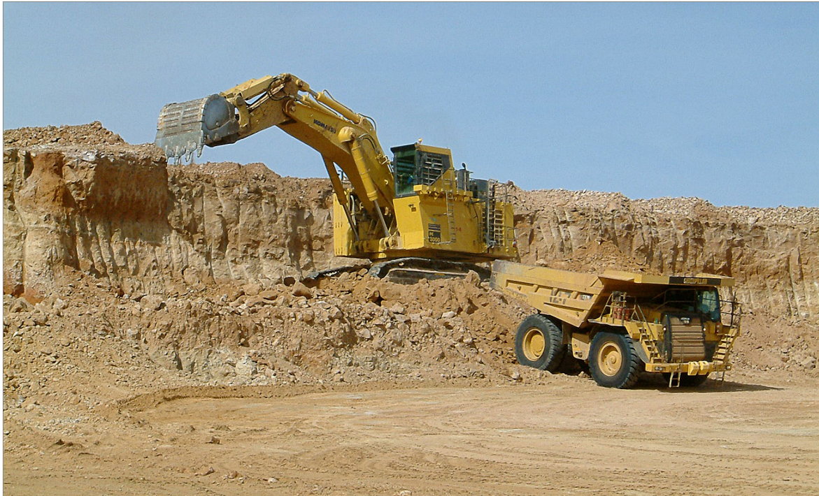
Figure 28: The unconsolidated ore sands at Brand se Baai are mined with front-end loaders in a load-and-carry operation. The hardened layers are mined using hydraulic excavators in a backhoe configuration or by trackdozer. Photo: BGR.
