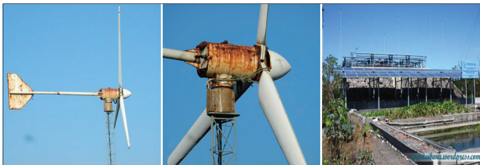
Figure 2: Corrosion in wind turbine and PLTH system
