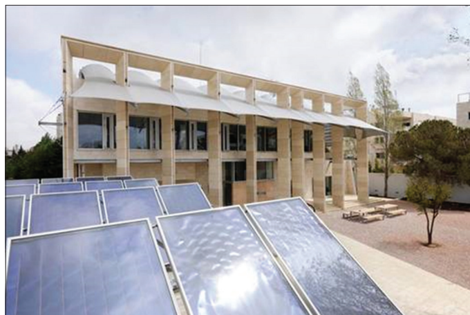
Figure 4: Solar thermal panels for hot water in the garden of the embassy
