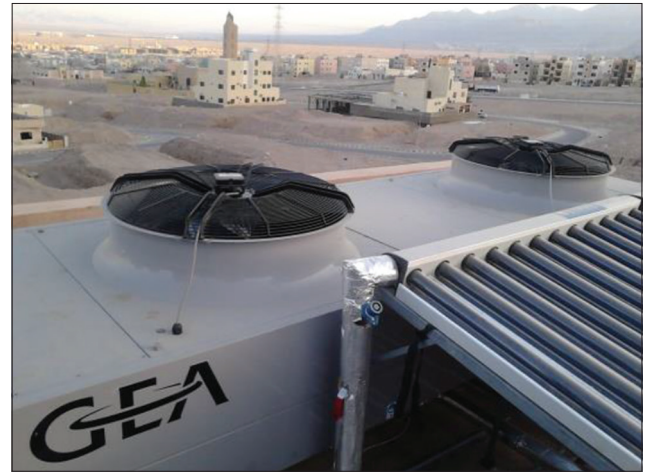
Figure 9: Dry Cooler installed at AR
