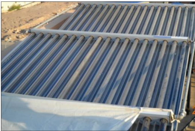
Figure 8: Solar water heaters installed at AR
