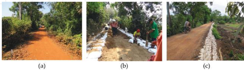
Figure 12. Construction of road embankment with Do-nou retaining wall: (a) Before construction; (b) construction of the embankment with Do-nou retaining wall; (c) after construction.
