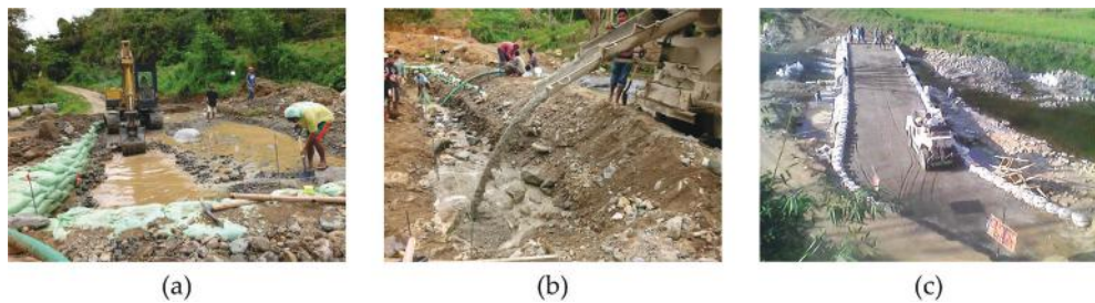
Figure 18. Work items managed using equipment provided by local government: (a) Excavation of the cut-off-wall and foundation; (b) transit mixers and water pump during casting concrete; (c) compaction of base course with roller.
