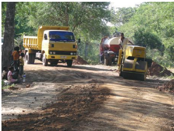
Figure 3. Road rehabilitation work in Timor Leste, using the equipment required for LBT.
