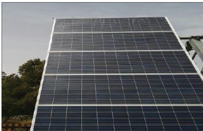
Figure 1: PV modules of nominal power of 285 Wp wired in series in one strings
