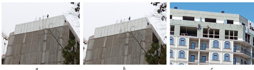
Fig. 1. Photo-fragment of application of the mixture: a – equipment adjustment; b – equipment cleaning; c – process of applying the mixture to a vertical surface
